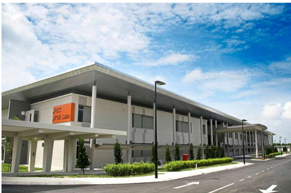
The exterior view of the Faculty of Information and Communication Technology (FICT) at the UTAR Perak Campus.
