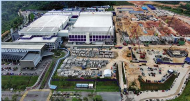
Infineon Kulim's expansion underway
