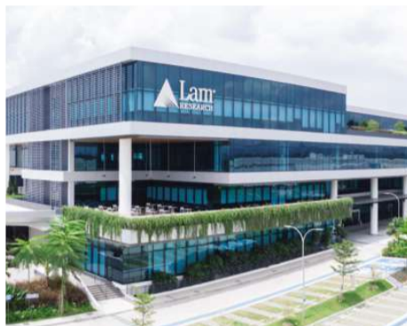
Lam Manufacturing Malaysia's state-of-the-art facility in Penang
