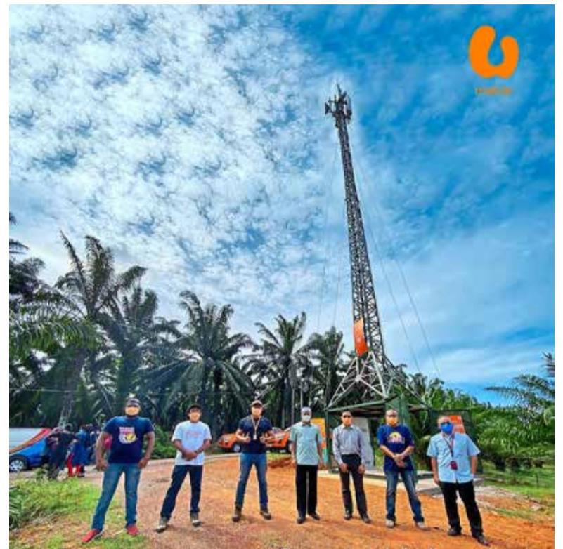
Temporary tower built in Kampung Kongs, Kedah to provide connectivity to the community.
