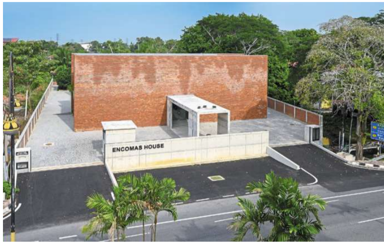
Over half of the external facade is made up of recycled clay bricks while the other half comprise plastered and glass walls.
