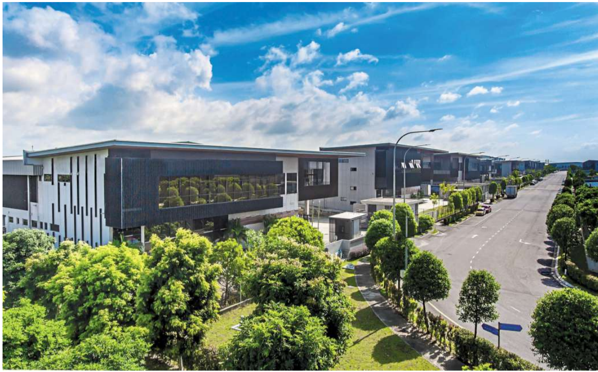
Lush greenery in overall development of i-Park@Senai Airport City.
