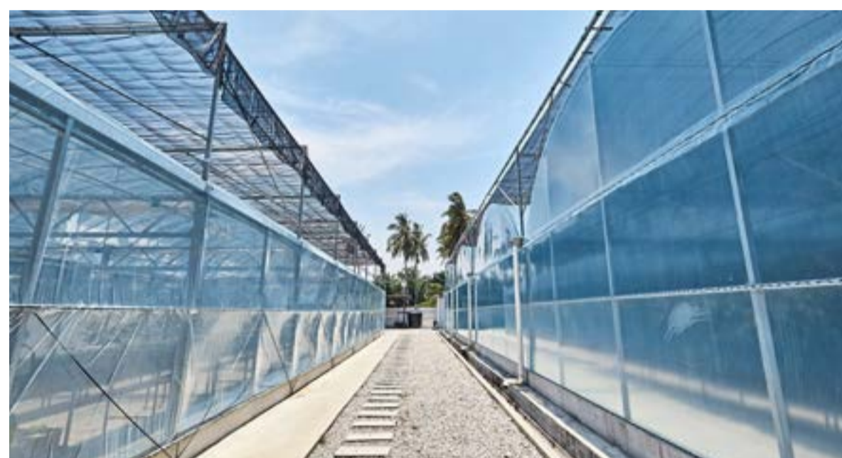
Semi-automated roofs adjust the amount of sunlight and heat into its greenhouses to maintain optimum environment for planting cool-weather crops.
