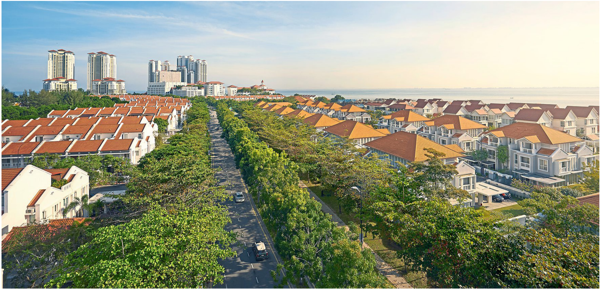
The second phase of the idyllic seafront township of Seri Tanjung Pinang in Penang is about to kick off, bringing more quality residential, commercial and leisure facilities.
