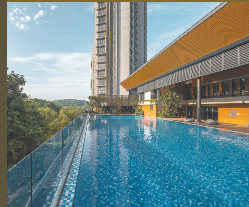
The Clio 2 Residences at IOI Resort City use a system formwork that uses prefab components to reduce material wastage, which is in line with IOIPG's Sustainability Policy and Waste Management Policy on using resources responsibly and minimising waste.
