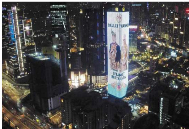
TSLAW Tower is recognised by the Malaysia Book of Records as the first and only one with 360° LED building facade display.
