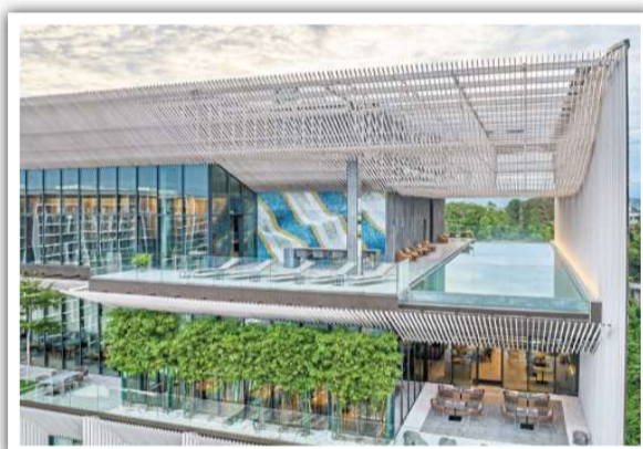
Double infinity edge swimming pool spatially extends towards Signal Hill and the South China Sea.
