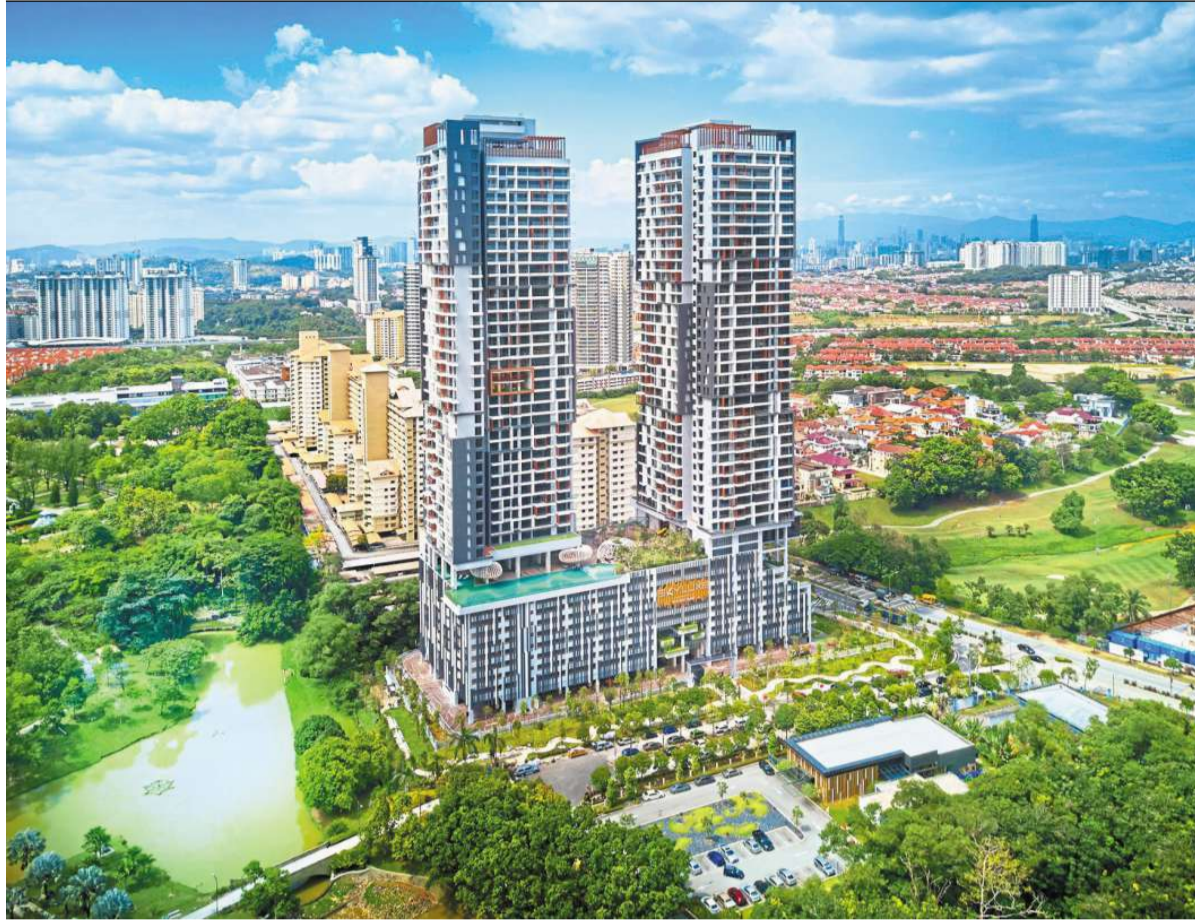
SkyLuxe on the Park Residences sets a new standard for urban high-rise living with its close proximity to Bukit Jalil's green lungs.
