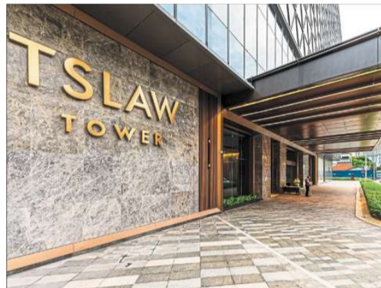
The building is the embodiment of corporate prestige with its grand design.
