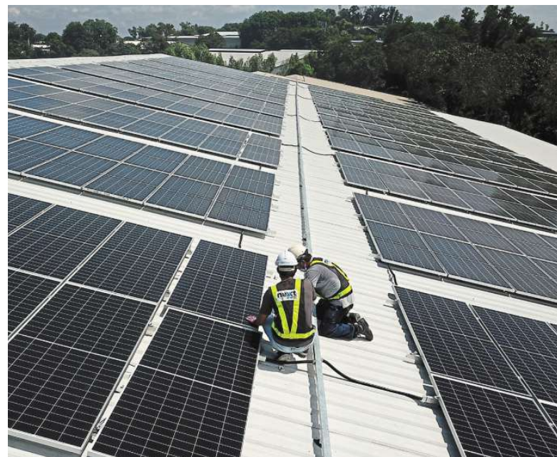
Next Energy is a trusted solar PV installer for residential, commercial, and industrial systems.
