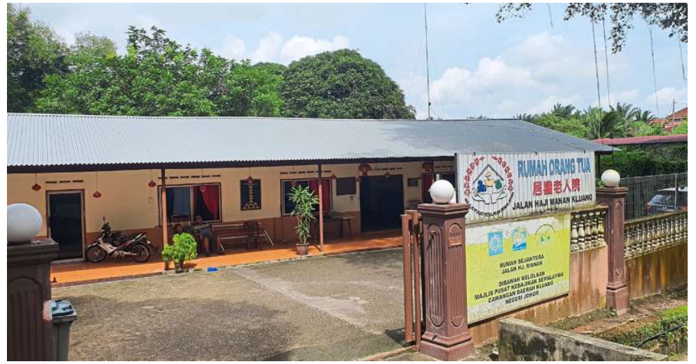
Colorbond Matt Steel by NS BlueScope Malaysia was used to fix the leaking and rusted roof at Rumah Orang Tua in Kluang.
