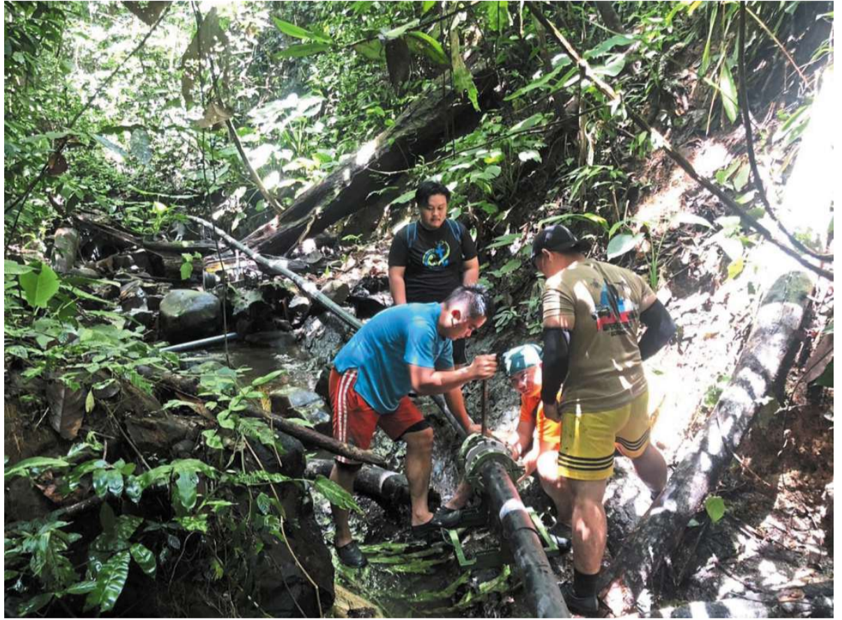
Villagers installing micro hydro pipes in their area.
