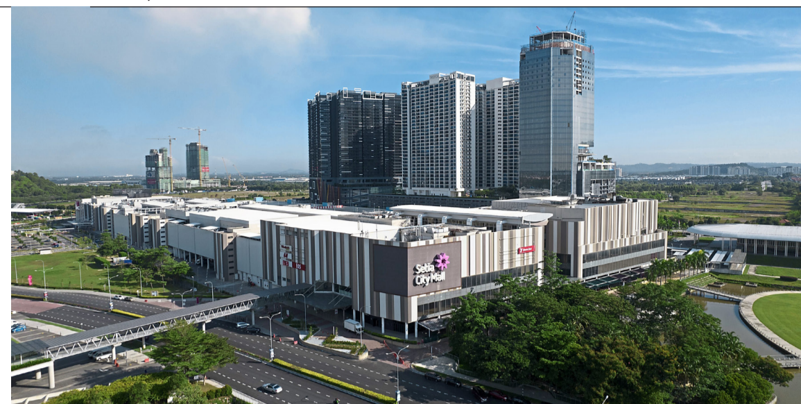
Setia City Mall in Setia Alam, Shah Alam.
